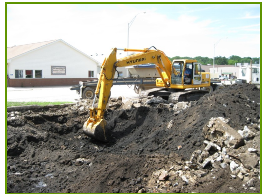
Remediation work at Winnebago Tribe of Nebraska
