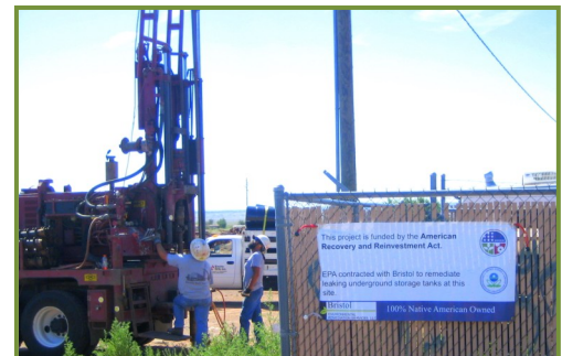
Remediation work at Navajo Nation, Arizona
