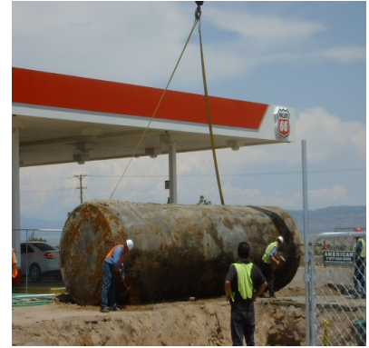
Remediation work at Domingo Trading Post, Kewa Pueblo, New Mexico
