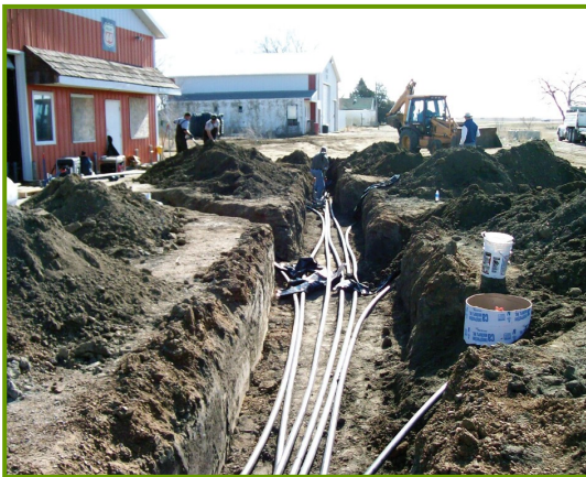
Remediation work on Cheyenne River Indian Reservation, South Dakota
