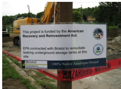
Remediation work at Winnebago Tribe of Nebraska
