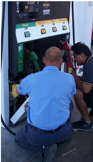
UST system operation and maintenance: examining a dispenser
