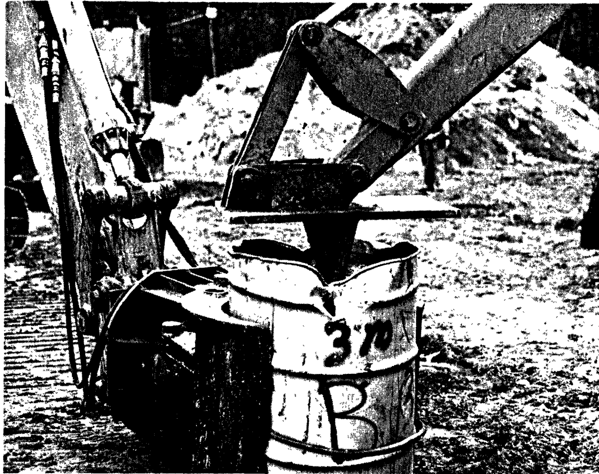
Figure 36. Backhoe Spike (nonsparking) Puncturing Drum Held by Grappler (Courtesy of O.H. Materials Co., Findlay, OH)
