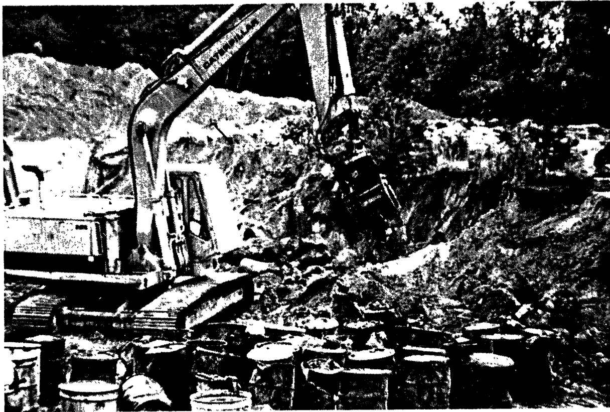
Figure 11. Barrel Grappler Removing Drums from Pit Excavation
