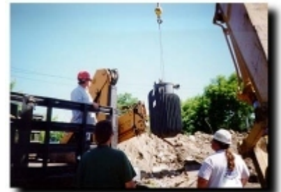
Transformers are removed from the Lily-Tulip site
