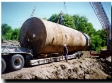
Underground storage tank removal
