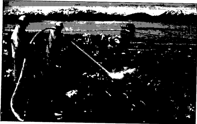
Response crews using high pressure hose to wash an oilcovered beach.
