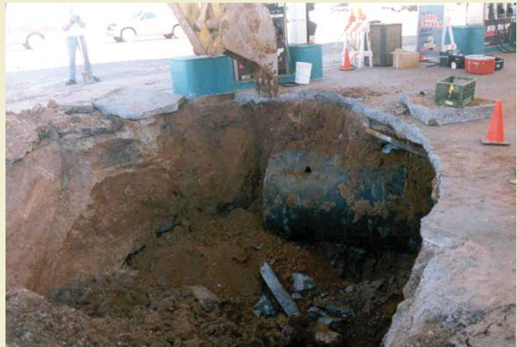
Lower right: Removal of leaking UST and contaminated soil.
