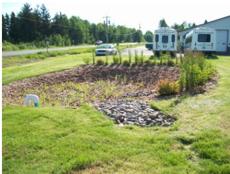
A "rain garden" has been established in this catchment for overflow runoff.
