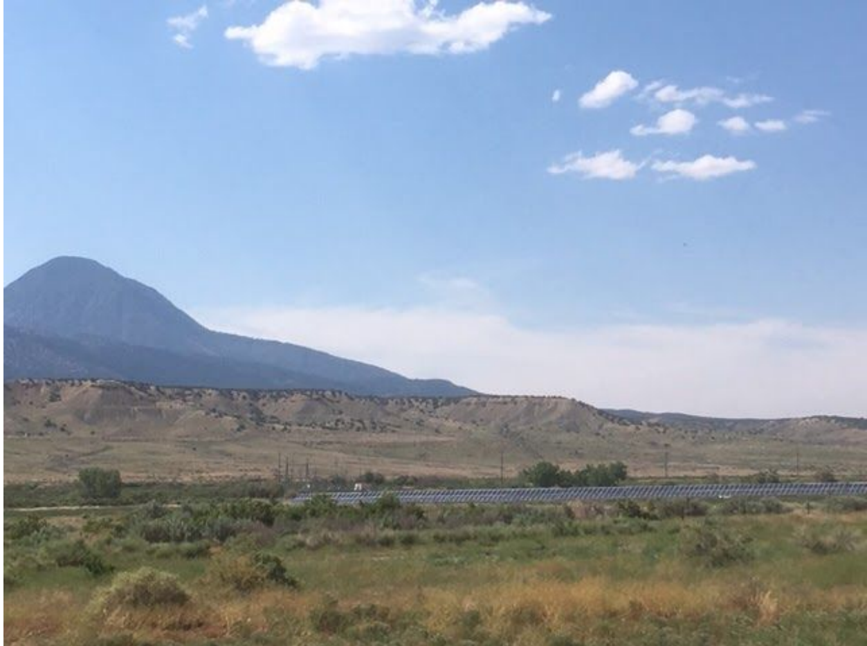
Towaoc Community Solar power plant - over 3800 PV panels, creatively net-metered, Ute Peak in background
