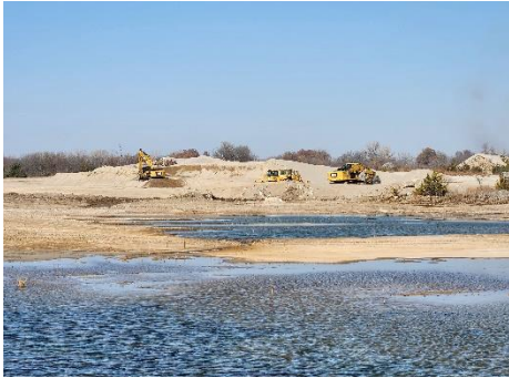
Ongoing remediation and restoration (Quapaw Nation)
