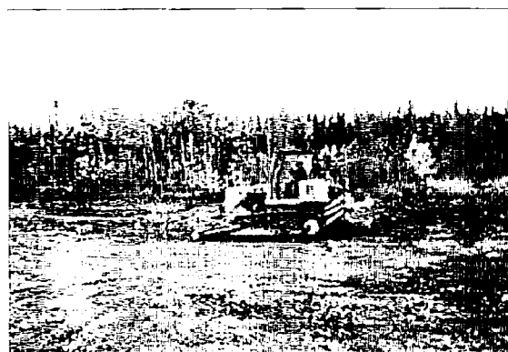
Bulldozer being used to consolidate, compact and cover waste at the landfill.
