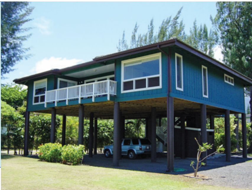
The FEMA flood zone in some areas on the north shore of Kaua‘i requires structures to be built at a minimum elevation. Credit: Dennis Hwang
