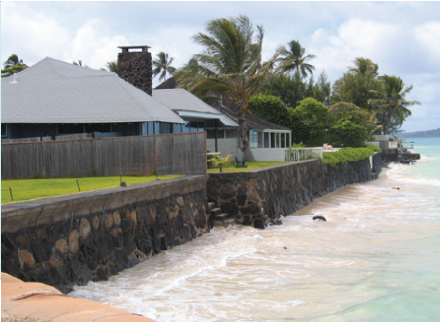
Regional armoring due to long-term chronic erosion has resulted in the loss of sandy beach in Lanikai, O‘ahu. Credit: UH Sea Grant
