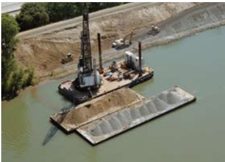
Levee repair site on Sacramento River
