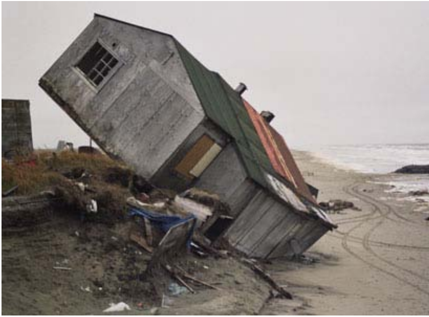
Coastal erosion led to the collapse of this house in Shishmaref, a Native Alaskan community that is seeking to relocate due to increasingly severe coastal disturbances. NPS Photo.
