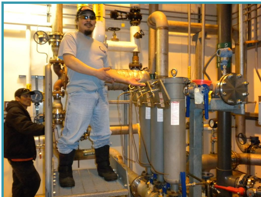
Fig. 1 Operator Andy Frankson at bag filter bank Photo M. Brubaker
