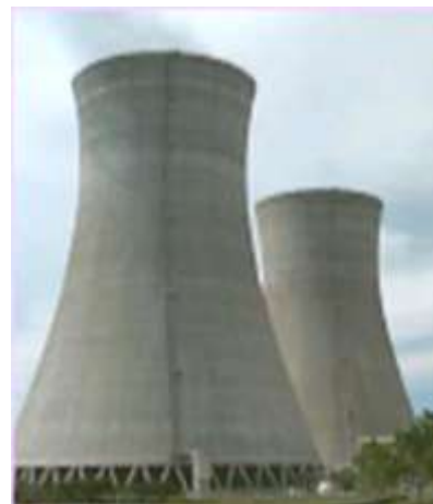
Figure 64 - Use of reclaimed water for cooling two 1 gigawatt plants in Miami-Dade County can use a total of 70-90 MGD of cooling water.
