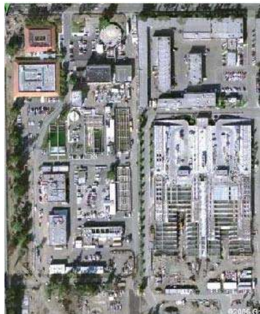
Figure 69 - Orange County, California Factory 21 Advanced Wastewater Treatment and Groundwater Replenishment.
