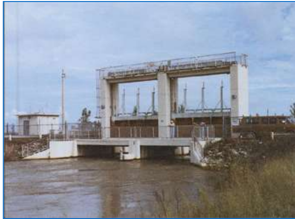
Figure 51 - Salinity structures control flooding by releasing primary canal water to tide when necessary. They are also used to maintain elevated canal levels for stormwater storage and to recharge aquifers and control saltwater intrusion. (SFWMD)
