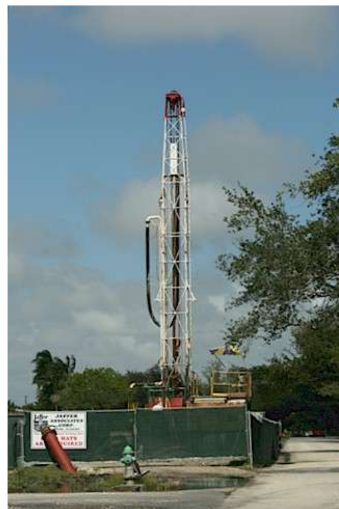
Figure 52 - Water well drilling rig
