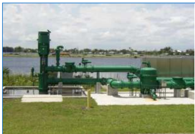
Figure 59 - A typical ASR well head.
