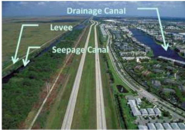
Figure 21 - The urban area is separated from the Everglades Water Conservation Areas by a levee. A seepage canal captures water the seeps under the levee. Drainage canals throughout the urban area maintain water tables and control flooding.
