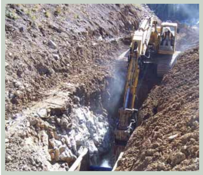
Construction of the Summitville Mine Hydroelectric Project's penstock.
