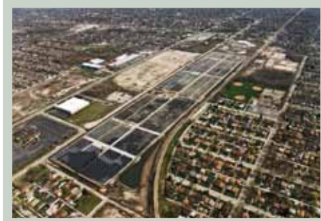
Aerial photographs of the Exelon City Solar Project pre- and post- construction
