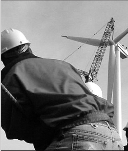
Raising the nacelle at Spirit Lake. Courtesy: Spirit Lake Community School District
