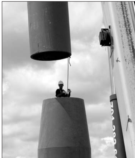
Setting up the White Earth wind tower. Photo credit: Nellis Kennedy
