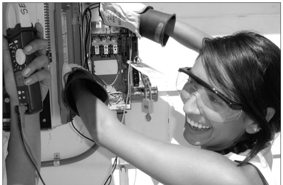
Honor the Earth Intern Yana Garcia working at a solar installation. Photo by Tom Reed.
