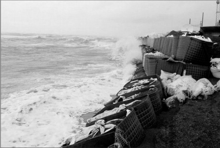
Waves pounding against the sandbagged seawall in Kivalina, Alaska. Photo credit: Mary Sage/AP
