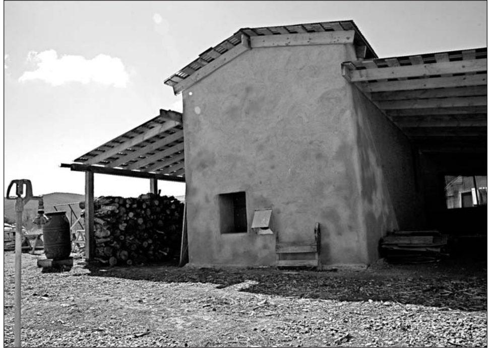
The GARN system has good potential to be replicated in Native communities and can heat a cluster of houses in a tribal community, as well as a single facility.
