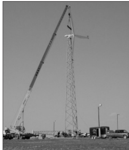
Erecting the Fort Peck turbine. Courtesy: Fort Peck Tribes
