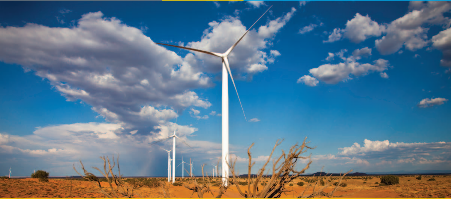
A WPA anemometer loan led to the construction of the 63-megawatt Dry Lake Wind Power Project, Arizona's first utility-scale wind farm.
