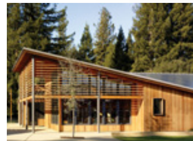
New library building with salvaged redwood siding and Alaskan Yellow Cedar sunscreen louvers.
