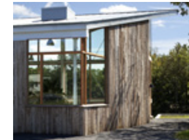
Reclaimed cypress wood siding came from mushroom farms.
