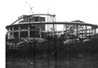
Original Palmer Auditorium under construction.
