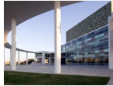
Aluminum panels from the original structure's dome added color to the Long Center's facade.
