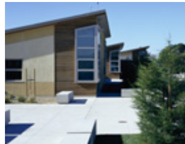
Classrooms clad with reclaimed redwood siding.
