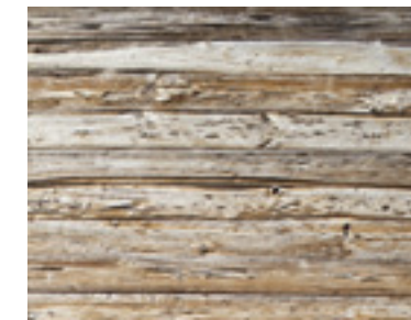
Exterior siding detail.
