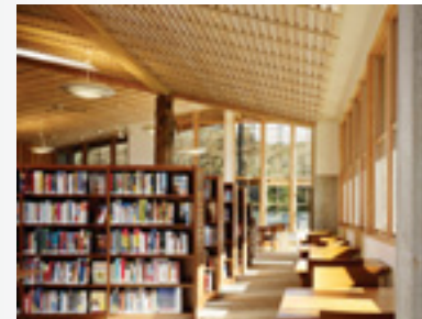
Interior of library building with salvaged wood ceiling paneling.
