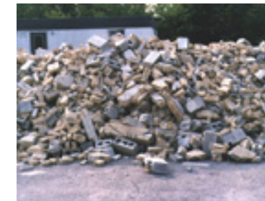
Concrete block from the original structure on the Ottawa site found new life in the exterior facade.
