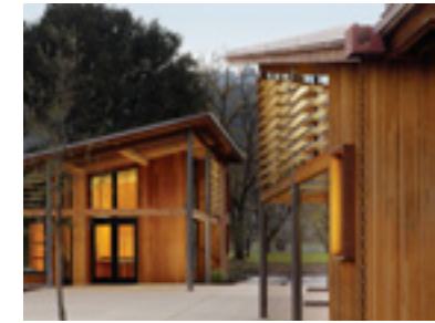
Portola Valley Town Center. Reclaimed Yellow Cedar was used to create sunscreen louvers. The buildings are clad in reclaimed redwood.
