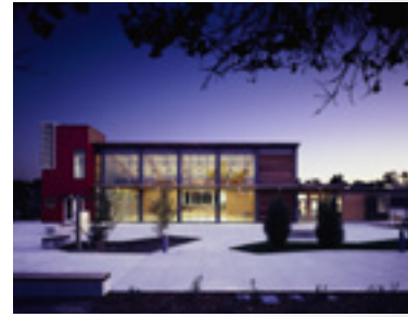
Chartwell School not only incorporates reuse, but thinks for the future by being designed for disassembly.
