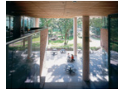
Reclaimed brick helps frame view to exterior courtyard.
