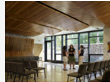
Ceiling paneling of reclaimed Cypress.
