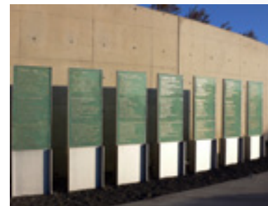
Glass curtain wall turned into donor panels.
