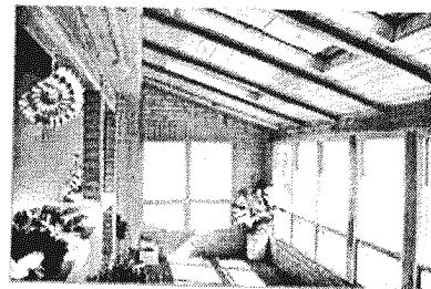
A sunspace or attached greenhouse relies primarily on convection to move heat from the sunny space to other adjacent rooms. Photo credit: Donald Aitken
