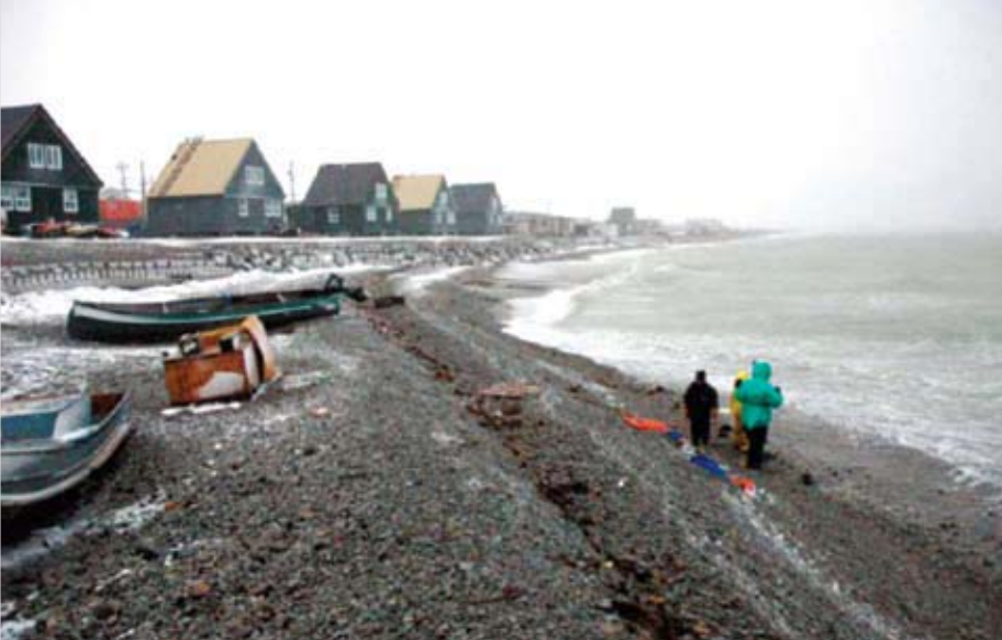
Examining erosion in Hall Beach, Nunavut
