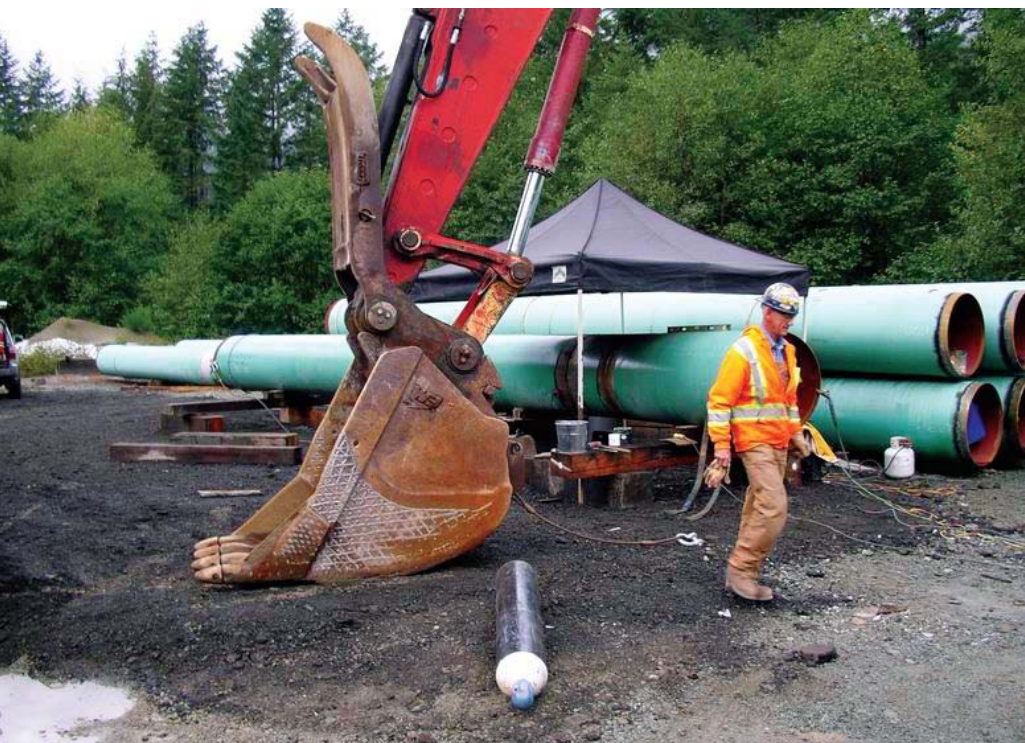
Construction of Canoe Creek Hydro Project Photo by: Tla-o-qui-aht First Nation
