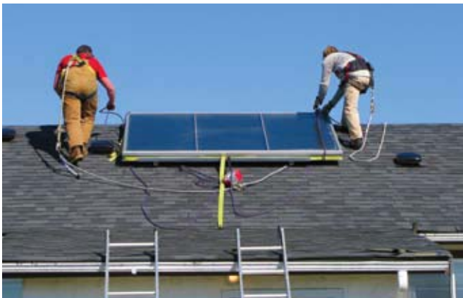
Solar Hot Water Panel Installation Photo by: T'Sou-ke First Nation
