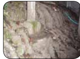
Visible erosion under a deck is common.
