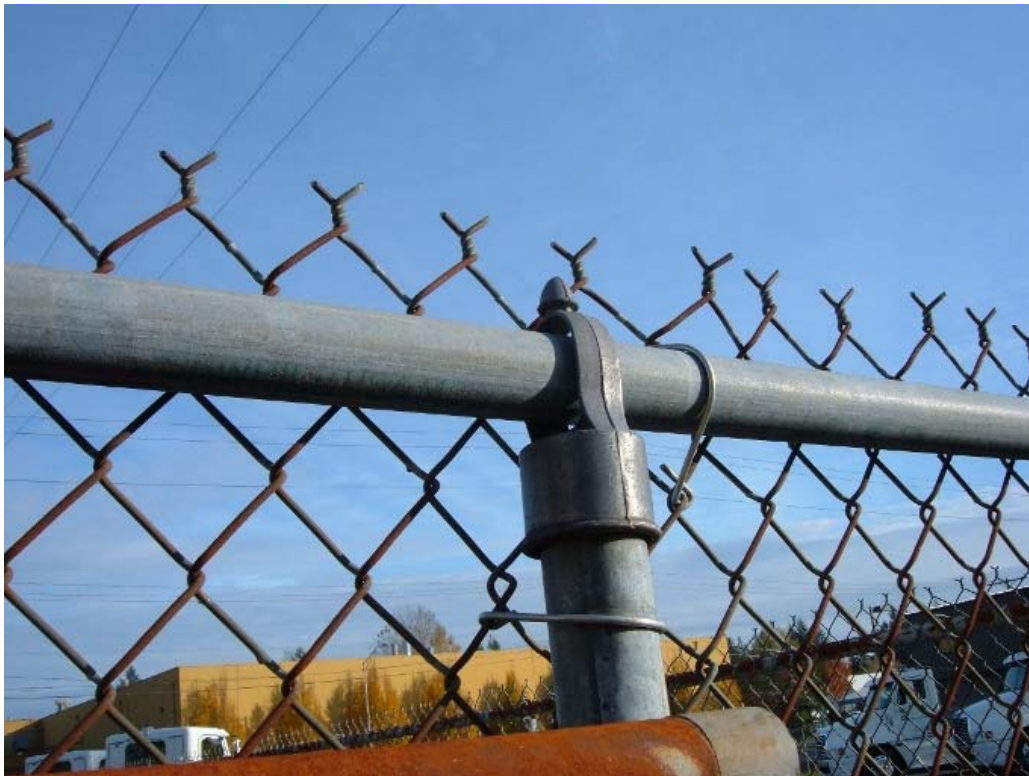
Galvanized chain-link fence can be a major source of zinc, especially when the fence is on paved rather than vegetated ground.
