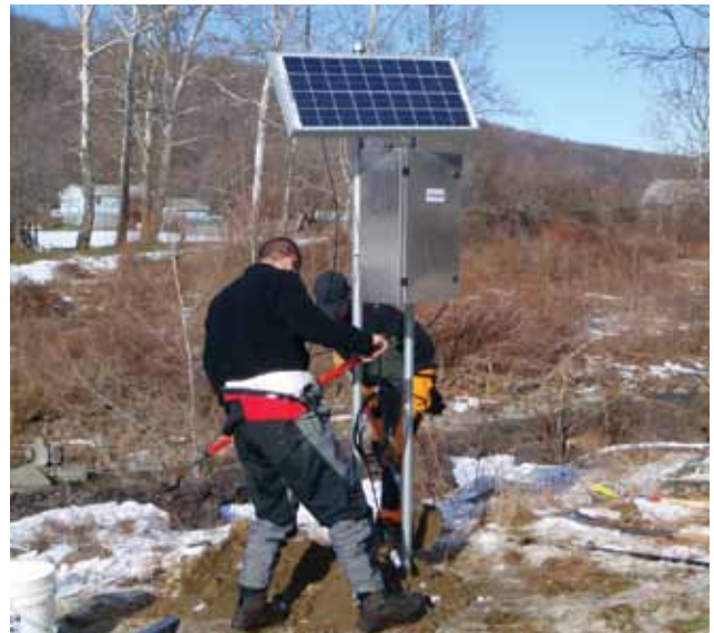
Jake Wilson (left) and John Balay of the Susquehanna River Basin Commission install a water quality monitoring station on Hammond Creek. (Photo: Andrew Gavin)
