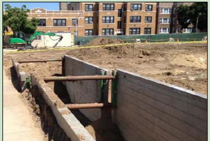
Mixing Trenches: At the Whitney Young Branch Library Brownfields Site, chemical oxidation reagents were mixed in three 16- by 16-foot trenches reinforced by steel. After mixing was complete, the steel was removed and reused onsite for purposes such as sidewalk shoring.
