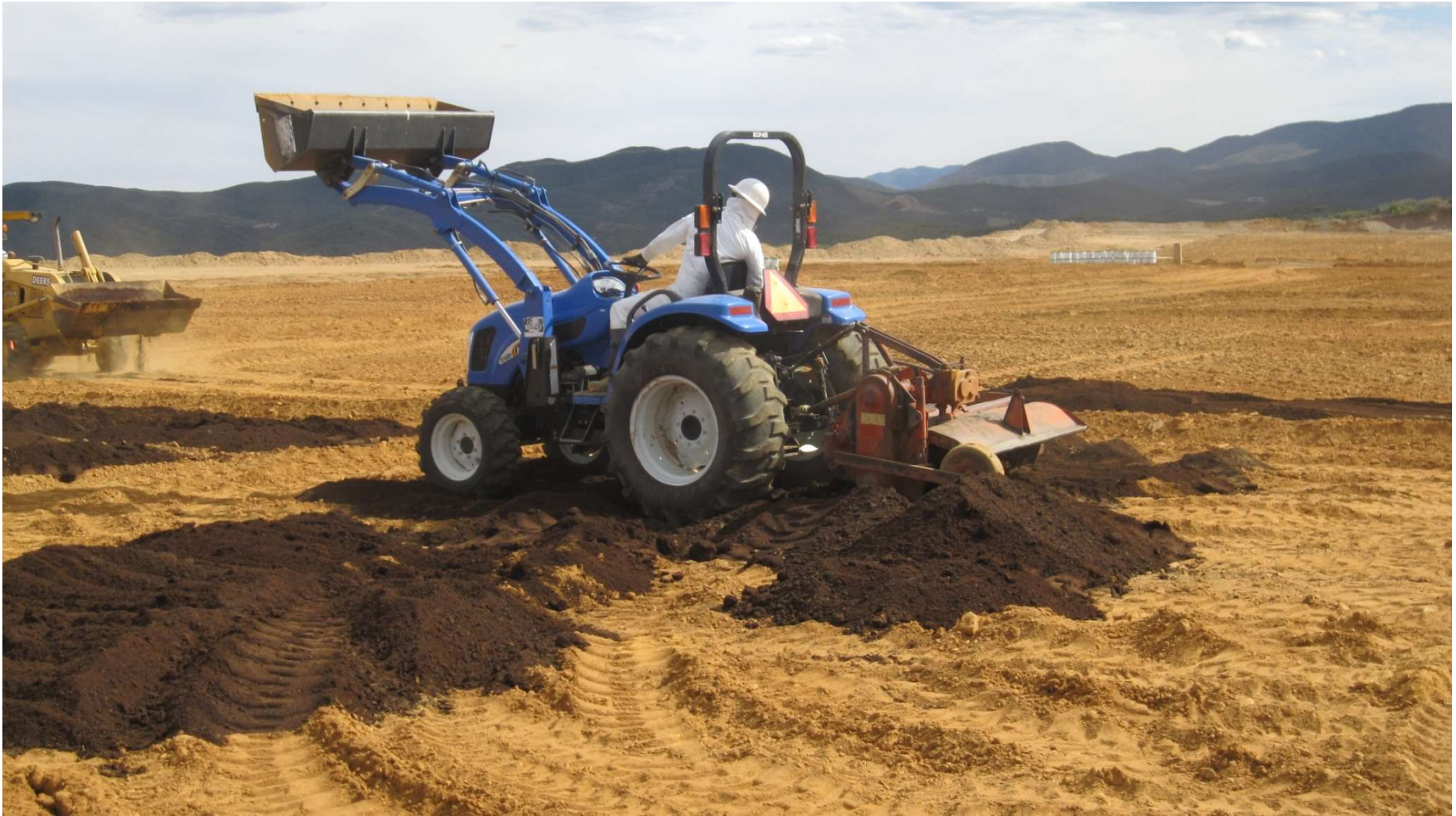
Mixing the compost into the tailings
