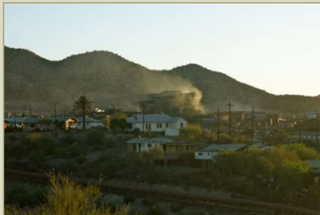
Hayden smelter building
