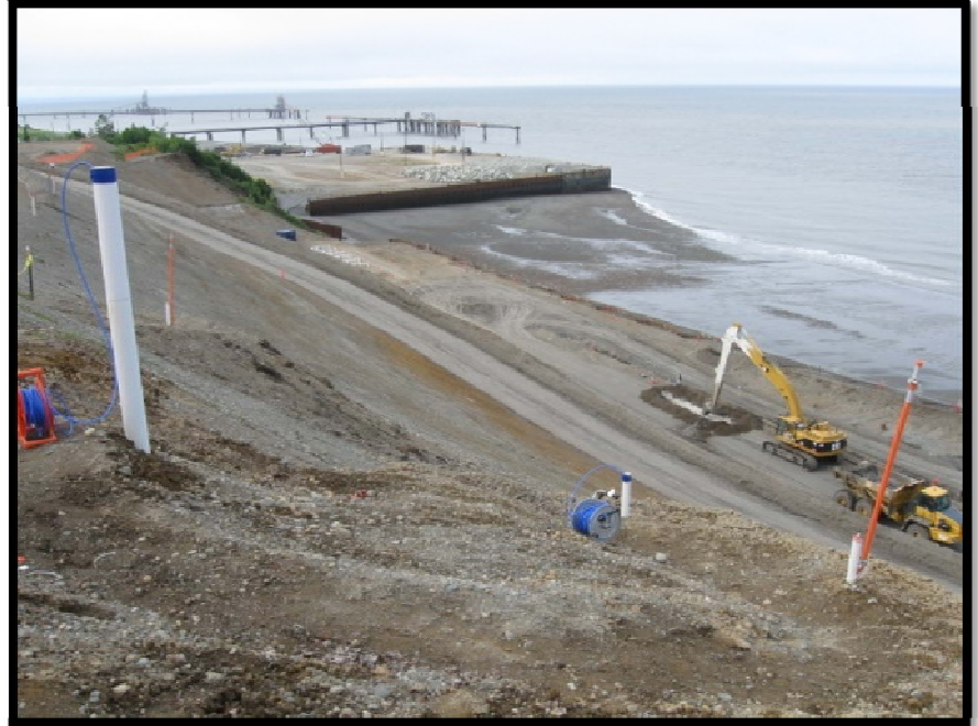
Installation of the slurry wall
