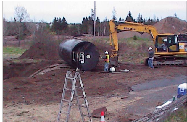
Tank removal activities at the Sipiyak Corner Store property.
