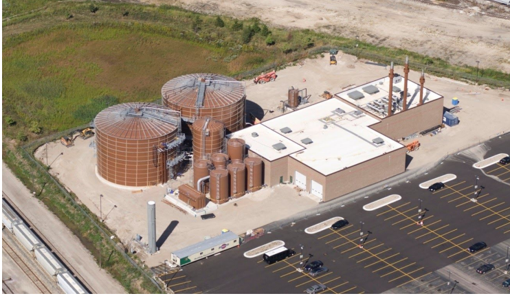
FCPC's biogas digester.
